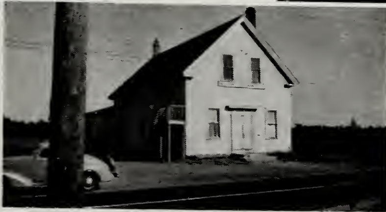
Top—LITTLE RED SCHOOL HOUSE Left—ASH DISTRICT SCHOOL Center—FIRST EAST SULLIVAN SCHOOL HOUSE Right—NORTH SULLIVAN SCHOOL HOUSE Lower—GRANGE HALL
